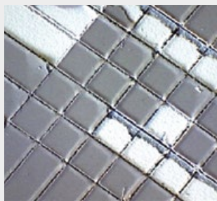
Loss of interlayer adhesion
